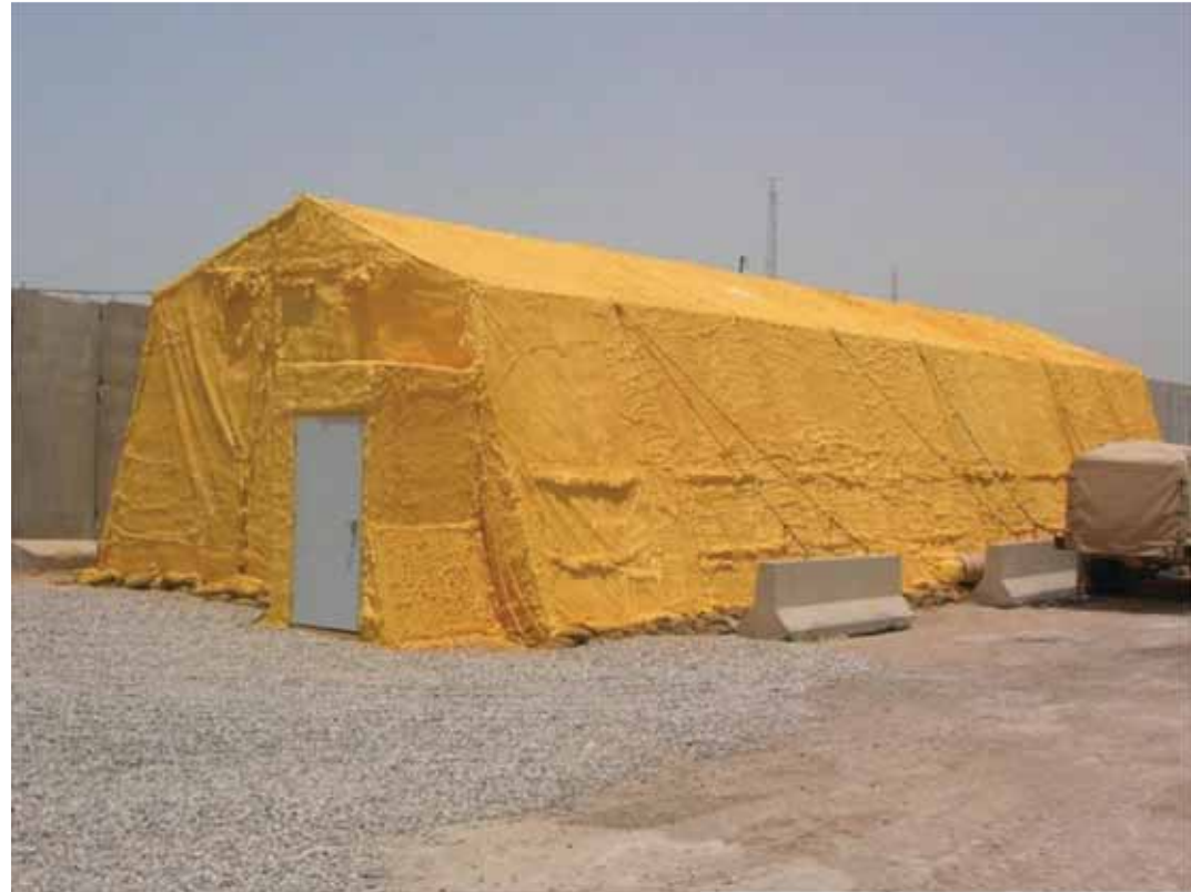
Spray Foam Insulation, Iraq
