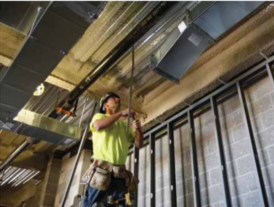
Tightly seal all joints at ducts
