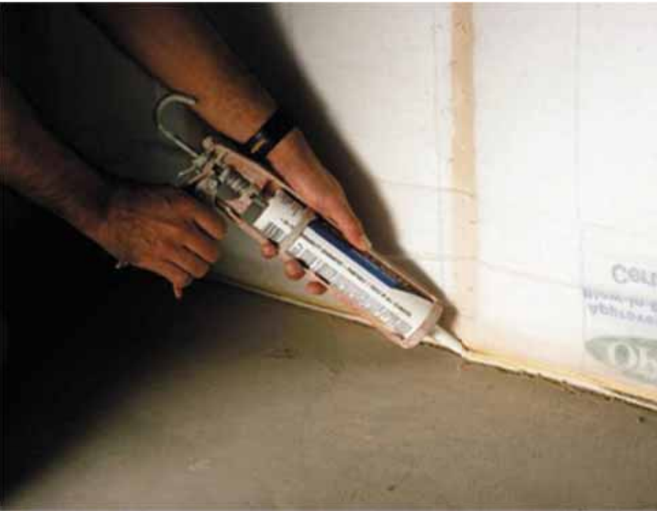
Air sealing with caulk
