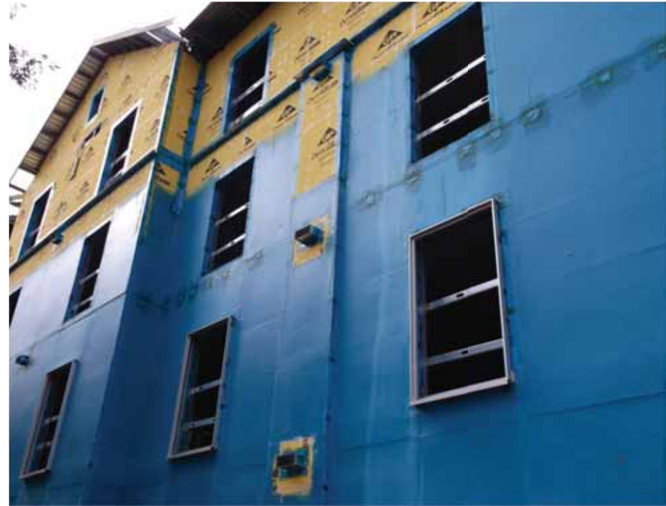
Liquid applied air barrier
