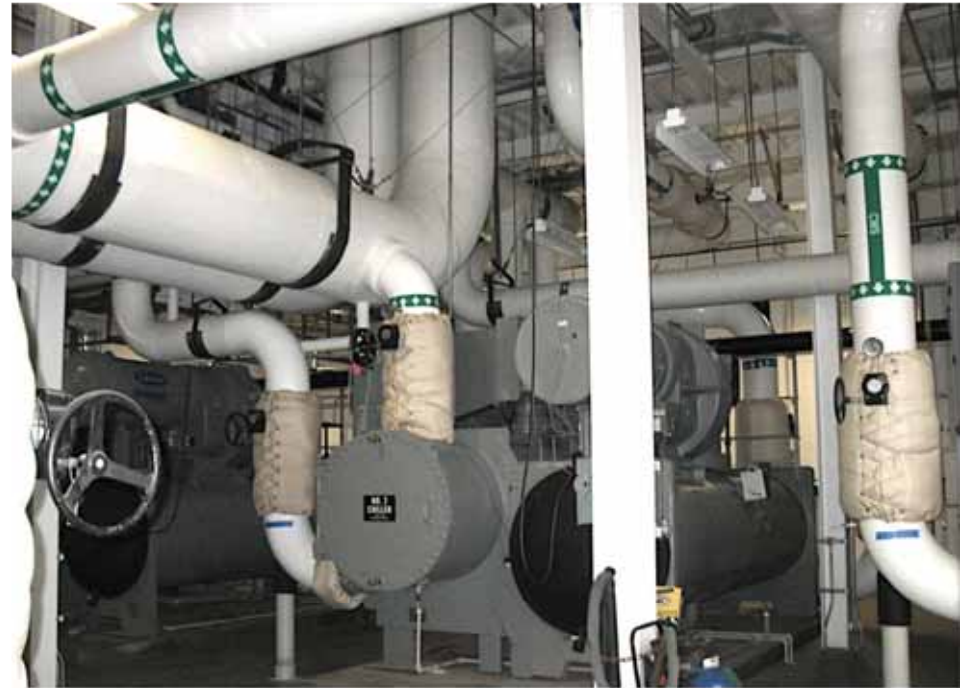
Insulate all pipes and ducts
